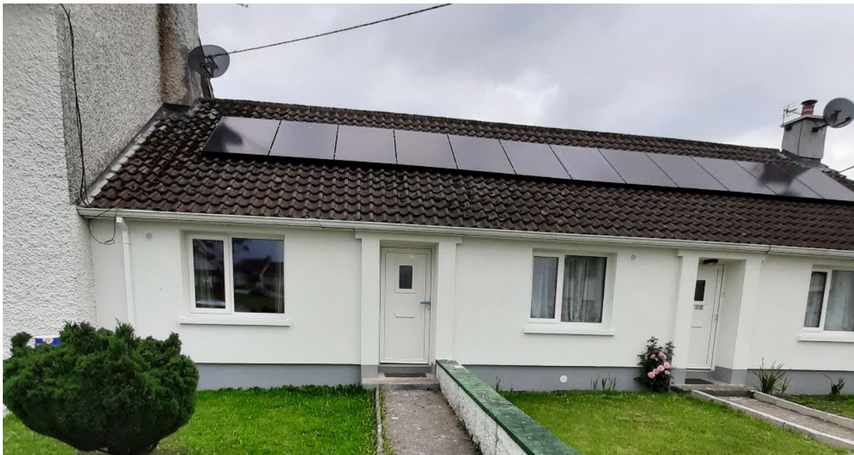
Photo of Energy Efficiency works including solar panels and air to water heat pump.
